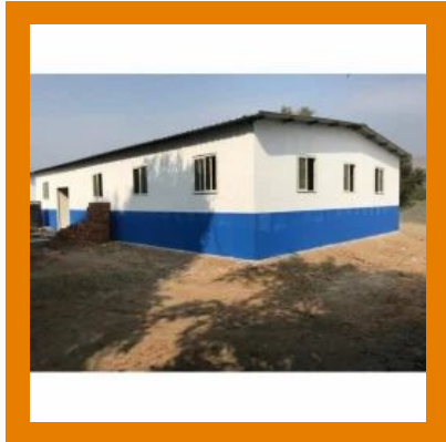
Prefab Class Rooms
