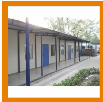
Workers Accommodation Structure
