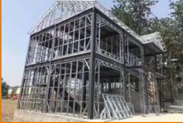
Prefab School Building
