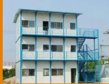
Prefab Staff Hutments
