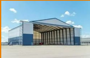
Temporary Storage Shed
