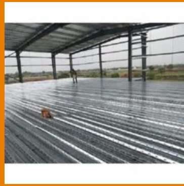
Mezzanine Decking Sheet
