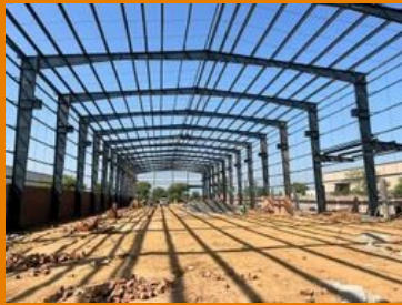
Pre- Fabricated Structures
